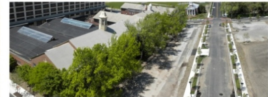
ROOF & PARKING LOT
